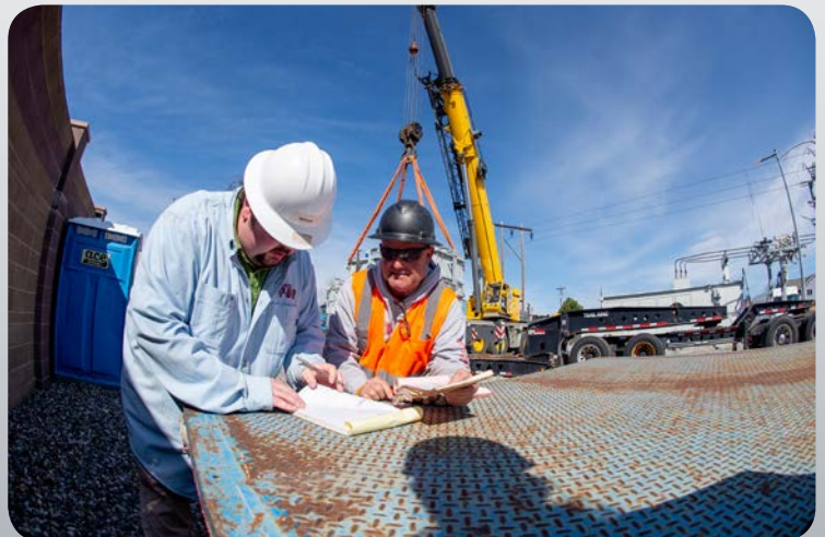
Installing new power transformer at the Orchard View substation.
