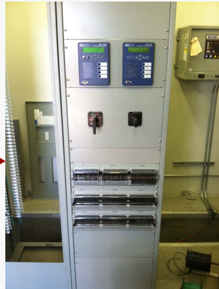
Protective Relay Upgrades
