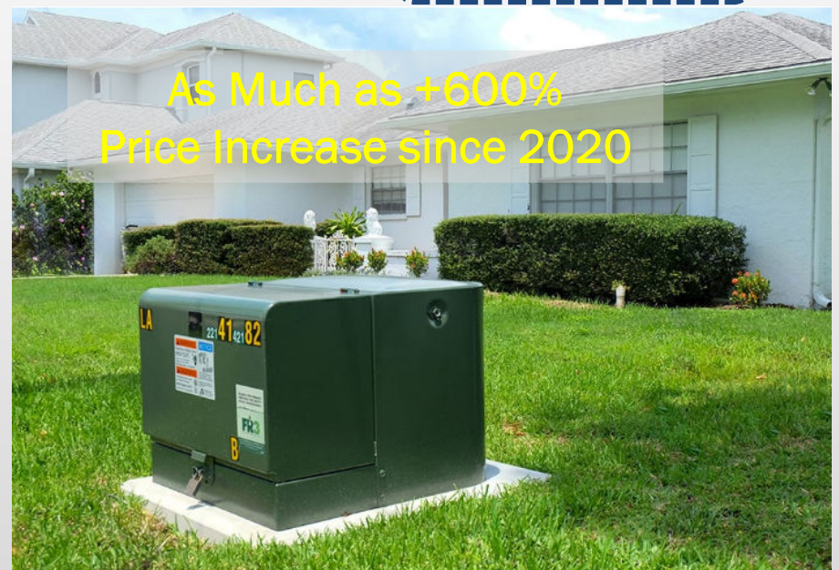
25-kilowatt Residential Transformer
